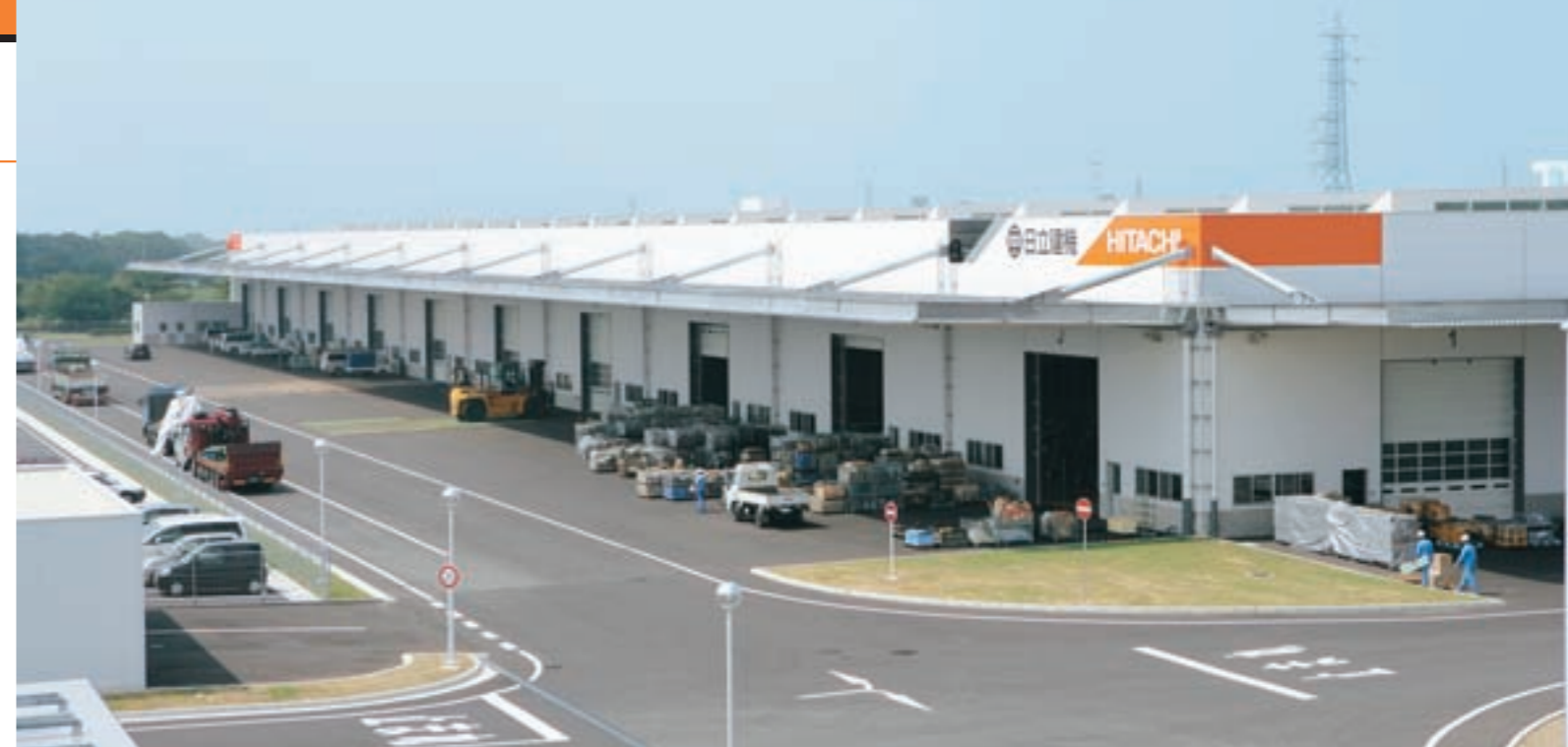
New plant appearance
