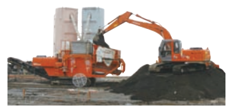
Soil remediation at site
