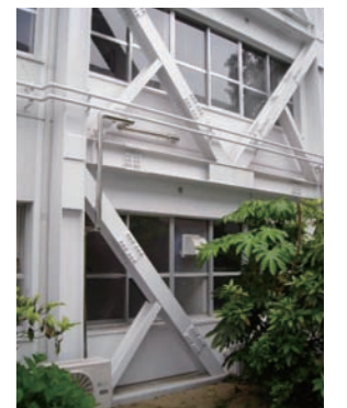
Tsuchiura Works East Building with earthquake reinforcement
